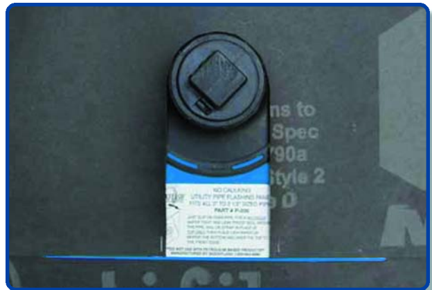
Plumbing Clean Out with QF Flashing Panel
