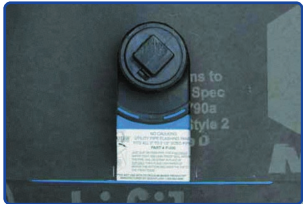
Plumbing Clean Out with QF Flashing Panel
