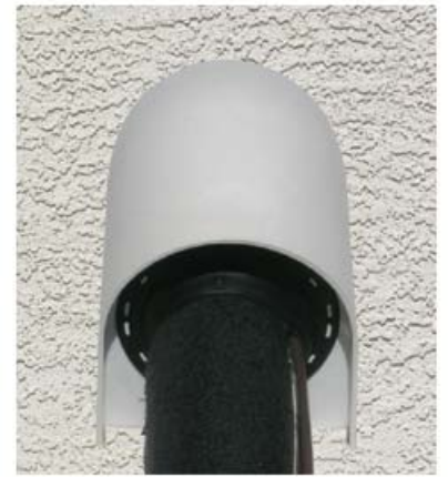
Recessed Seal w/ Drip Edge
